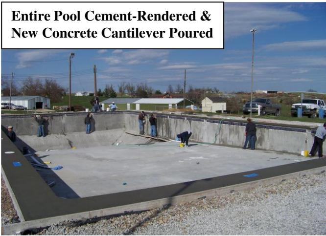
**Entire Pool Cement-Rendered & New Concrete Cantilever Poured**
