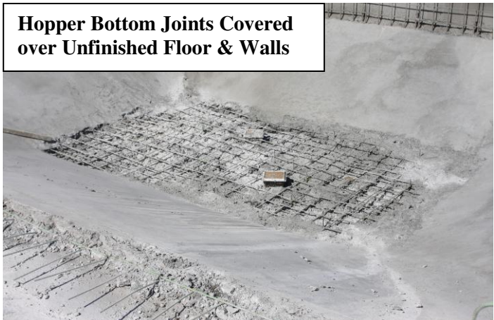
Steel Re-done and Confined to Cantilever Area
