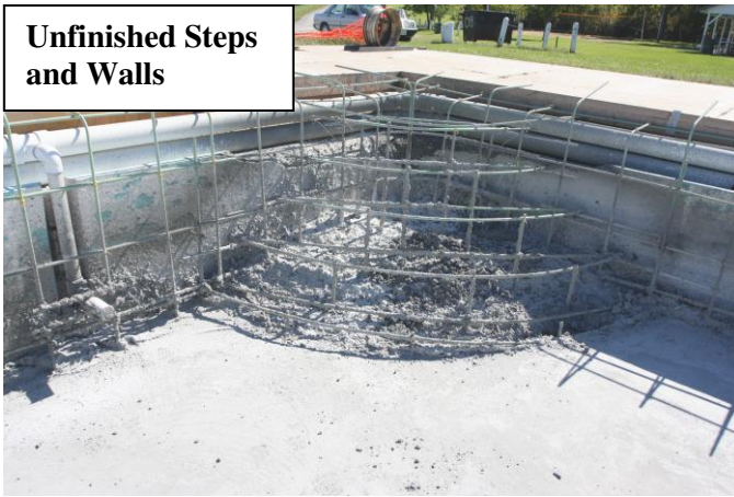
Steel Extending into Decking Area (Not Recommended)
