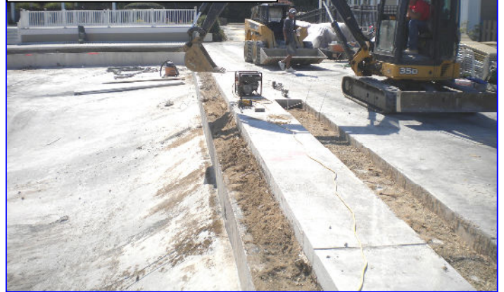
Top of Pool Cut for New Stainless Steel Gutters
