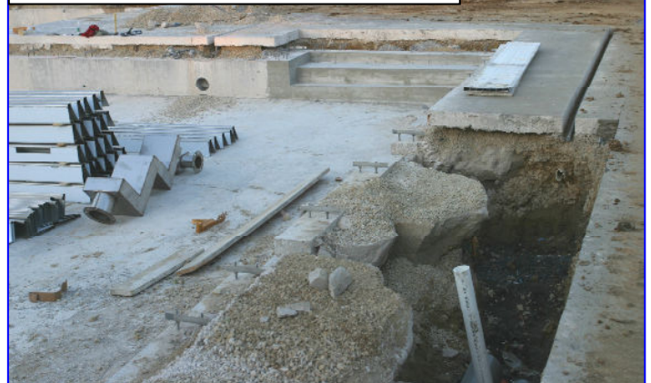
New Entry Steps Formed & Poured
