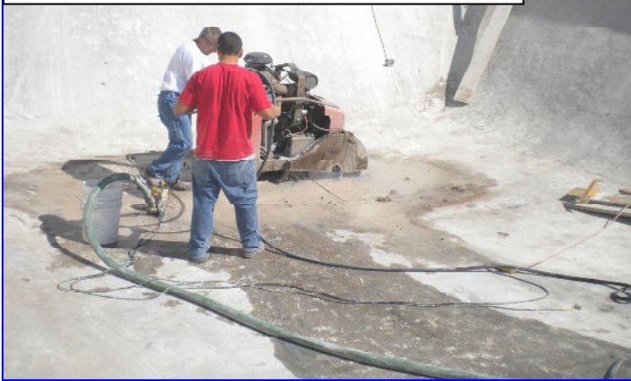
Saw Cutting for New Main Drain Sumps
