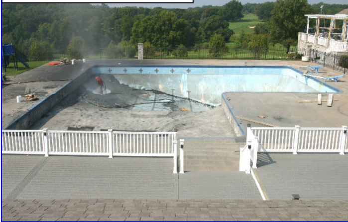
Paint Removal Underway
