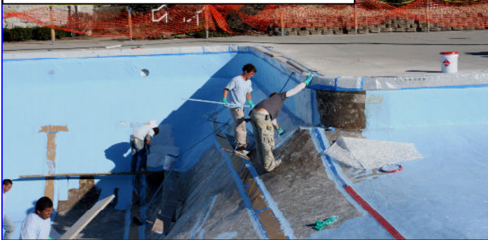
Installation of Blue INTER-GLASS® Two-Tiered Scaffolds for Depth
