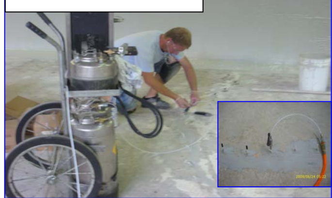
Epoxy Injection in Progress
