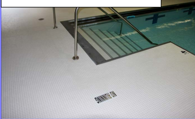
New Concrete Steps & Gutter Additions
