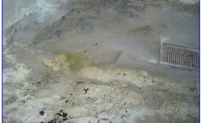
Surface Condition Found Under the Liner After Removal
