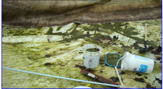
Liner Removal in Progress
