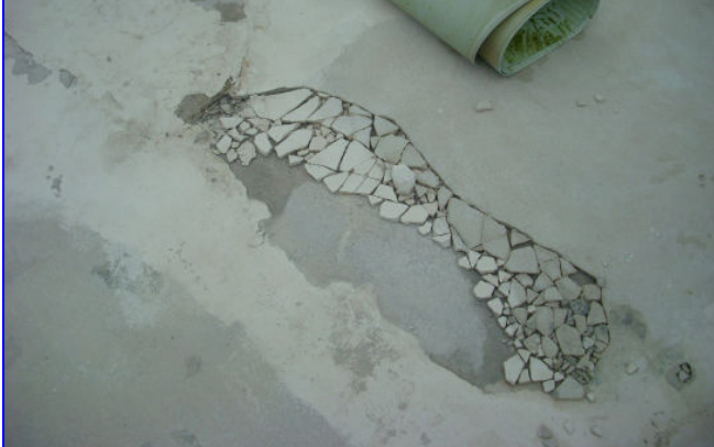
Effects on Concrete Under a PVC Liner from Freeze/Thaw Cycling
