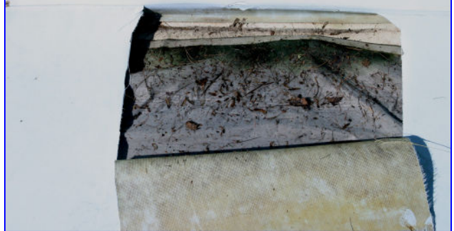
Surface Condition Found Under the Liner After Removal
