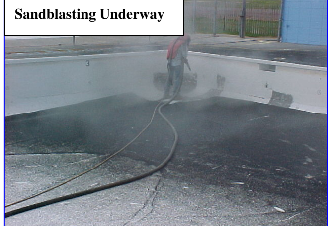
Concrete Removal Underway
