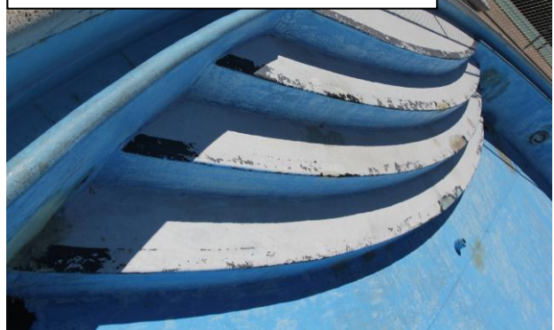
Entry Steps at Start of Project
