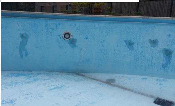
Surface Before Removal Begins
