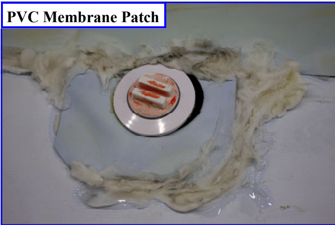
Pool Interior Patching After Removal
