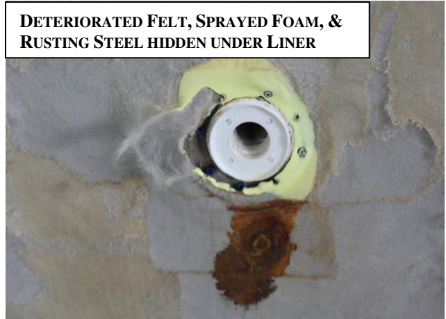
PENETRATING RESIN PRIOR TO INTER-GLASS® INSTALLATION
