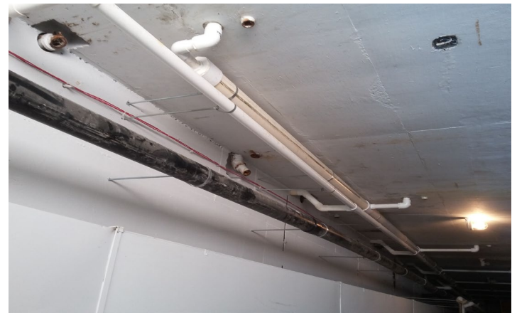
New PVC Recirculation Lines in Process of Installation
