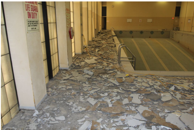
Thin Deck Membrane in process of Removal
