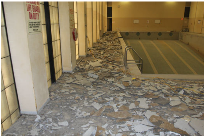
Thin Deck Membrane in process of Removal
