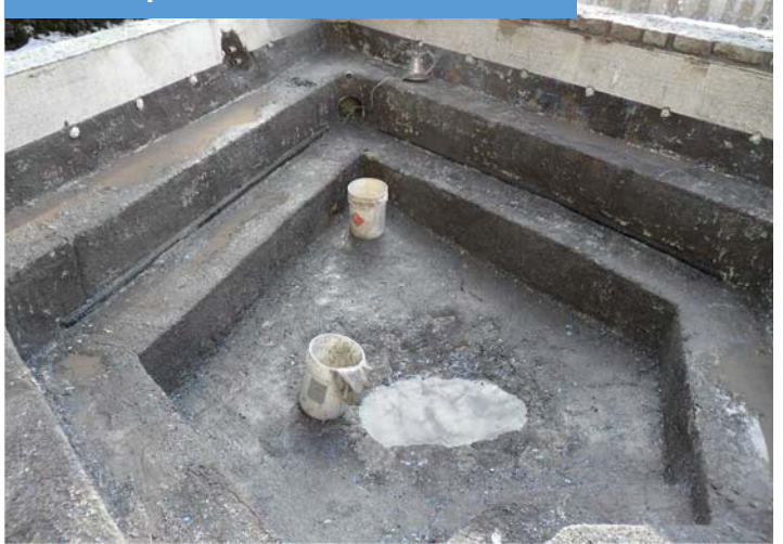
Gutted Spa to Sound Concrete Base
